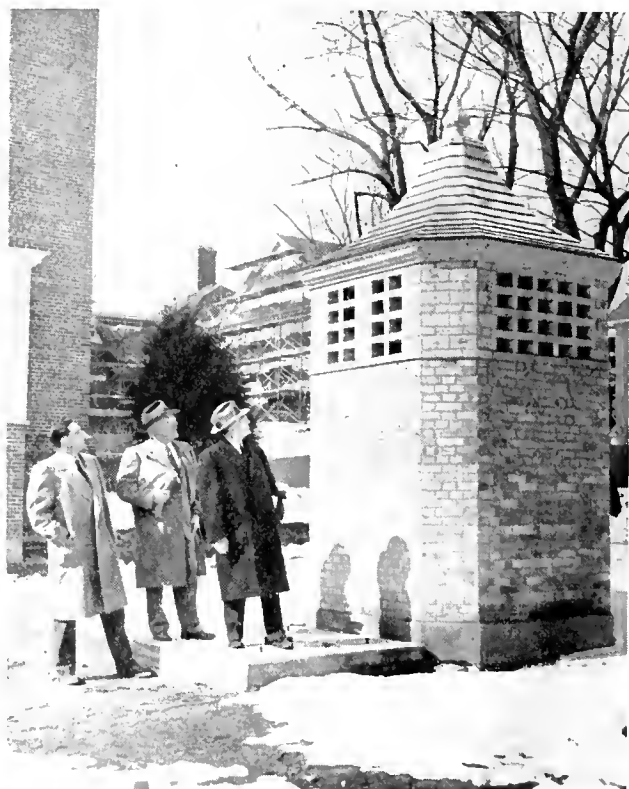
"WHAT IS IT?" The question is often asked in the Quadrangle. City ordinances require ventilators, with openings seven feet up in the air, over underground electrical transformers. To the architects, working in the Georgian, they posed a problem in style. Nearest counterpart is the "gazebo," a Colonial summer-house.
