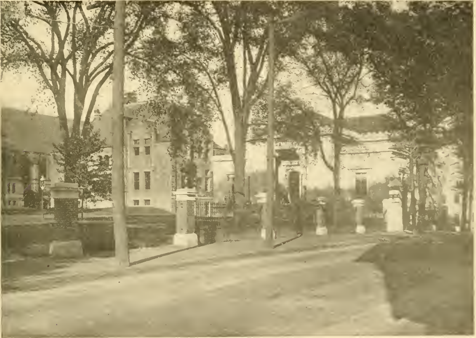
THE NEW FENCE ALONG GEORGE STREET
