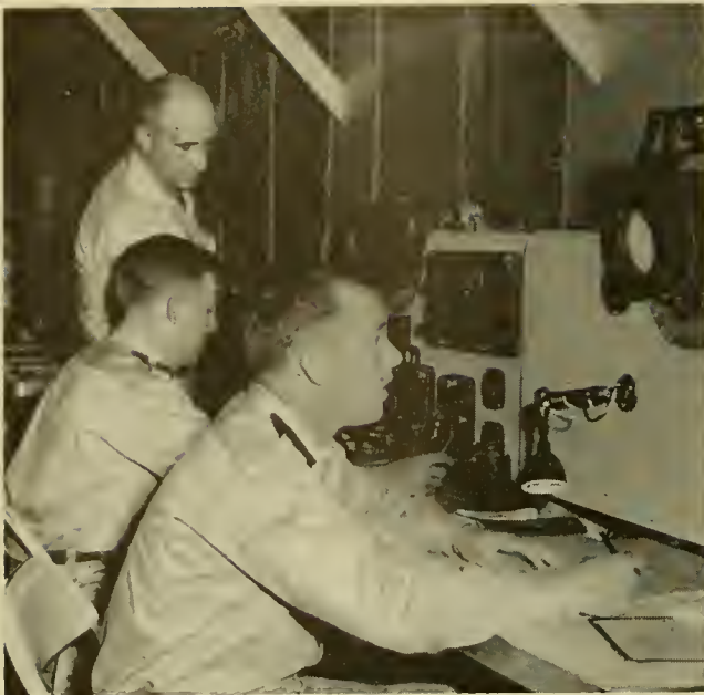
MOCK-UP of a navigation trainer lets the Cadets solve a problem such as would be encountered in actual flight. The radarscope projects map.
