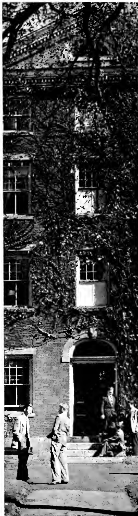
Its restoration will start this year.
