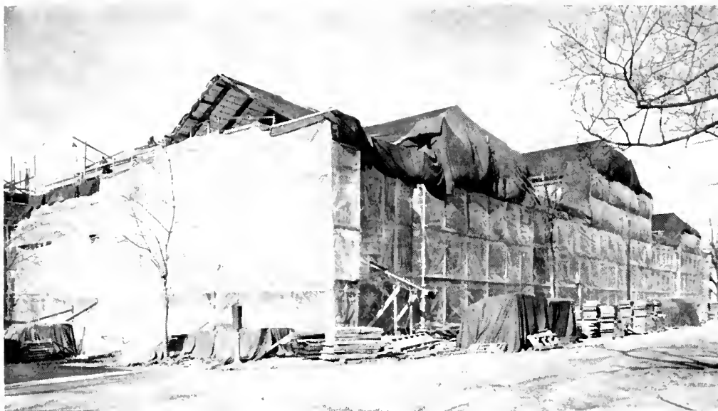
EVEN IN SUB-ZERO WEATHER, bricklayers could work inside the novel "plastic wrapping." The covering, believed one of the largest anywhere, provided a steam-heated corridor on the outside of the Quodrangle. View is from the southeast.
