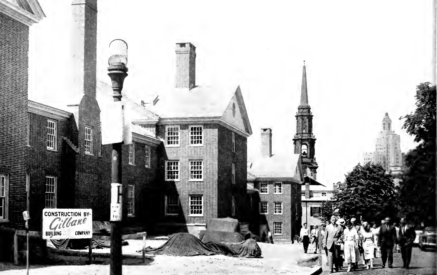
LOOKING DOWN Benevolent from Brown St. toward the City. Corner at left was site of the former Alumni House.
