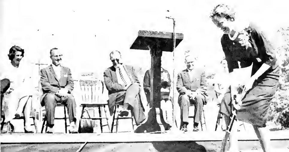
IT'S AT PEMBROKE as they break ground for the new dormitories there. . . .
