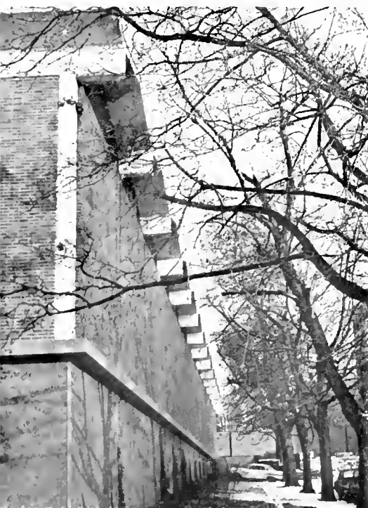
THE FLANK of the Prince Engineering Lab.
