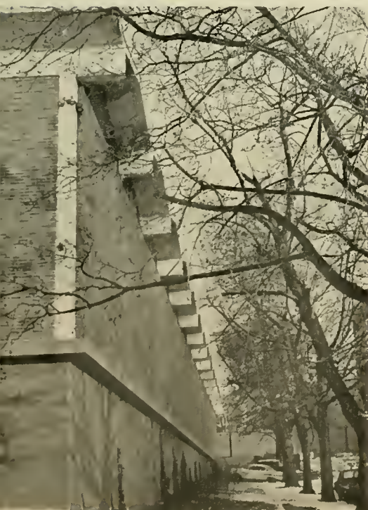
THE FLANK of the Prince Engineering Lab.
