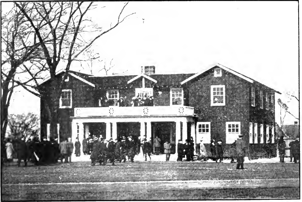
MARSTON FIELD HOUSE
