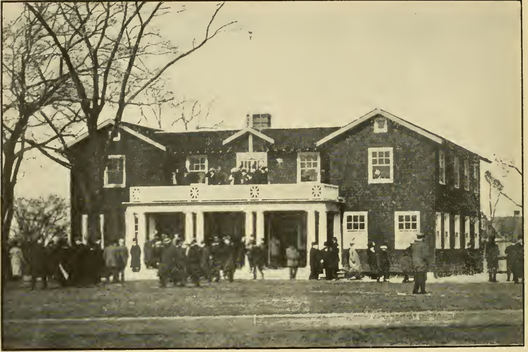
MARSTON FIELD HOUSE
