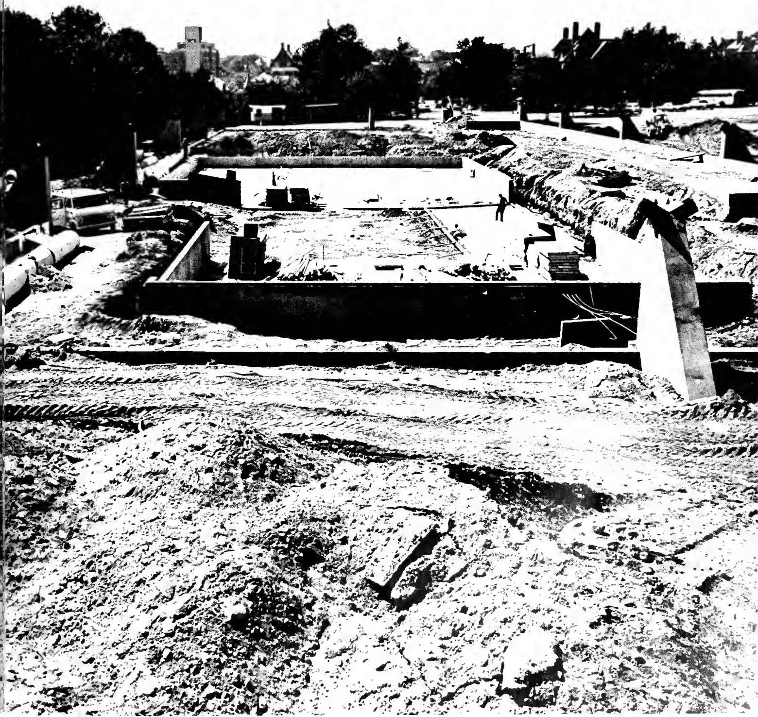
The construction site for the new swimming pool—looking west.
