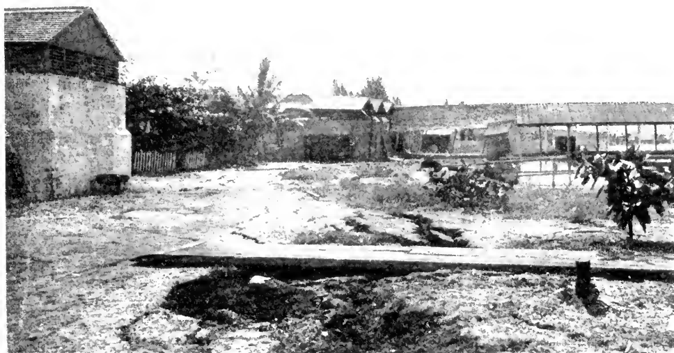
ZONE OF FISSURES IN THE PALISADOES. SHOWING SLIGHT SUBSIDENCE OF BUILDINGS
