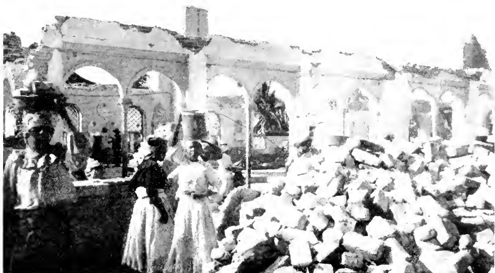
AT WORK UPON THE RUINS OF THE CATHOLIC CATHEDRAL. THE LINE OF ARCHES IS PARALLEL TO THE DIRECTION OF THE SHOCK
