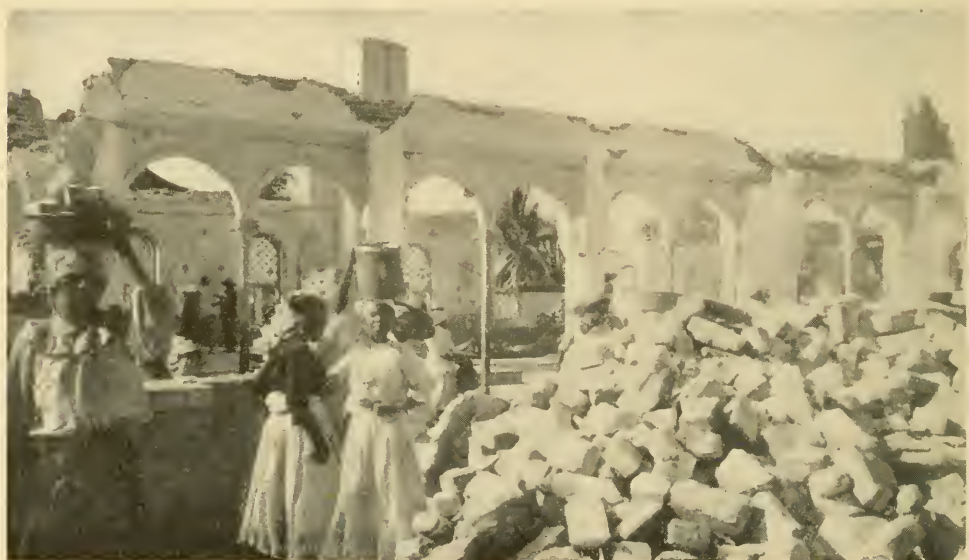
AT WORK UPON THE RUINS OF THE CATHOLIC CATHEDRAL. THE LINE OF ARCHES IS PARALLEL TO THE DIRECTION OF THE SHOCK
