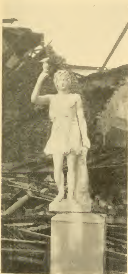
STATUE NEARLY TWISTED OFF THE PEDESTAL BY TWO COMPONENTS OF THE SHOCK
