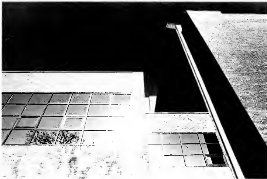
The new (left) rests against the old (right).
