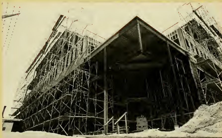
Construction of Brown's new multi-purpose Center for Information Technology proceeds on schedule.
