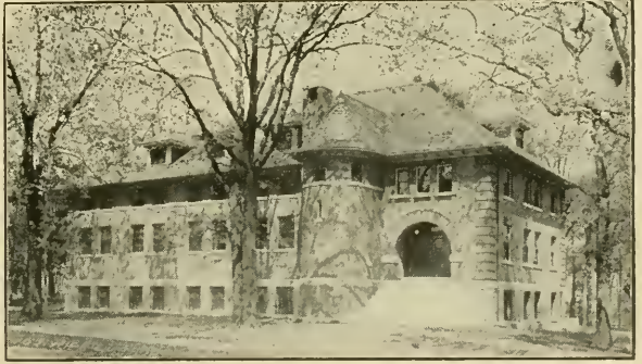
VIEW OF GYMNASIUM.
