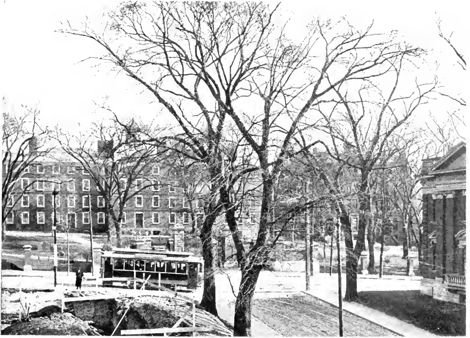
SHOWING EXCAVATIONS FOR JOHN HAY LIBRARY
