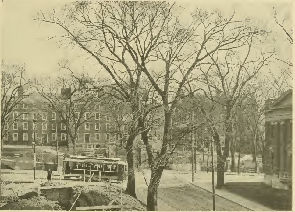
SHOWING EXCAVATIONS FOR JOHN HAY LIBRARY
