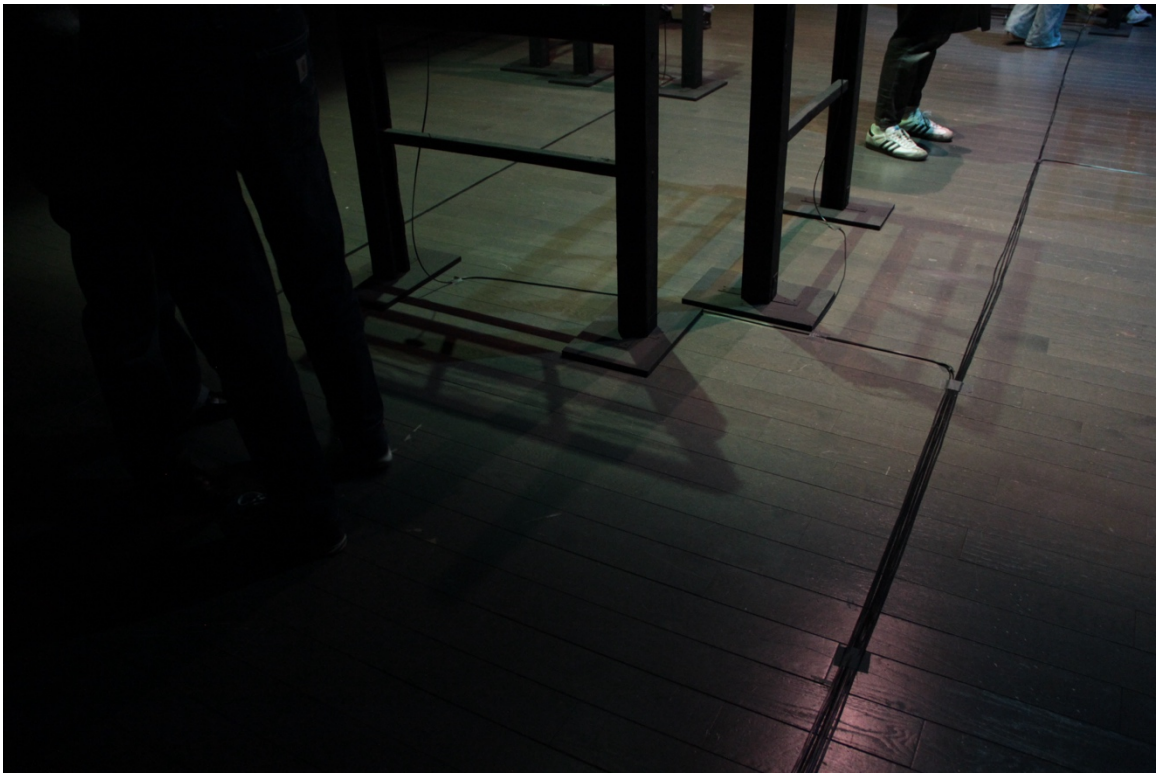
Figure 5: Cables running from each window and joining the flow towards the monitoring station.
