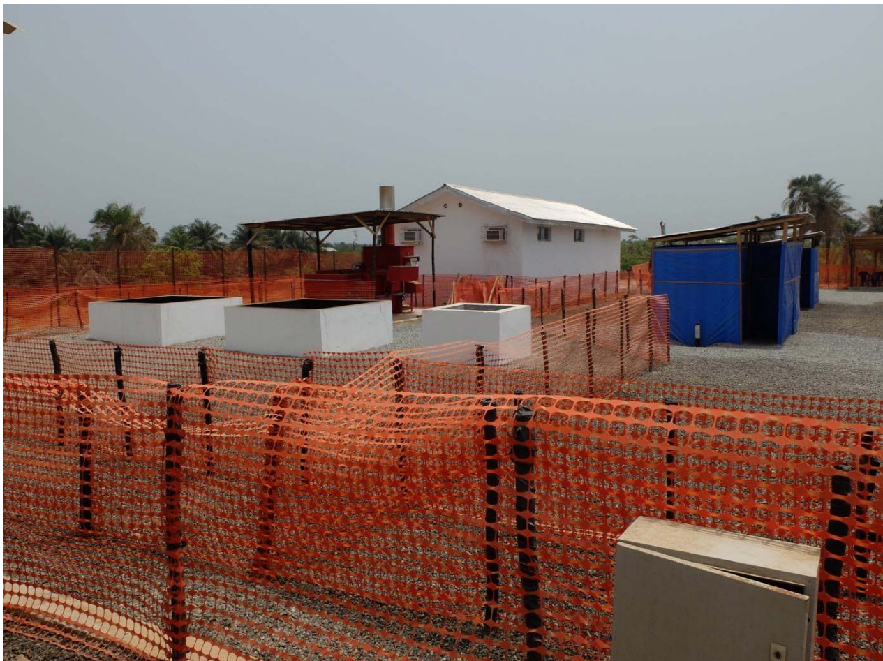
The incinerators within the unit. All contaminated material was daily buried by Guinean paramedics, 2015. Photo: Veronica Gomez-Temesio.
